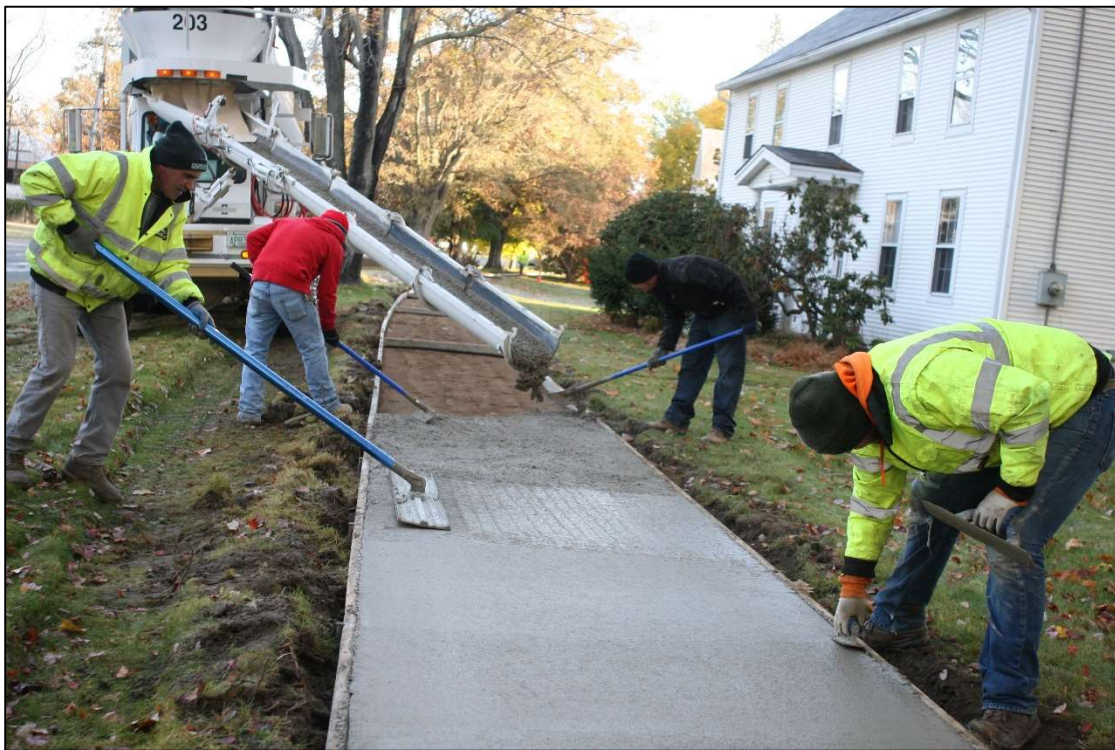
Hatfield DPW installing sidewalks on Main Street.
