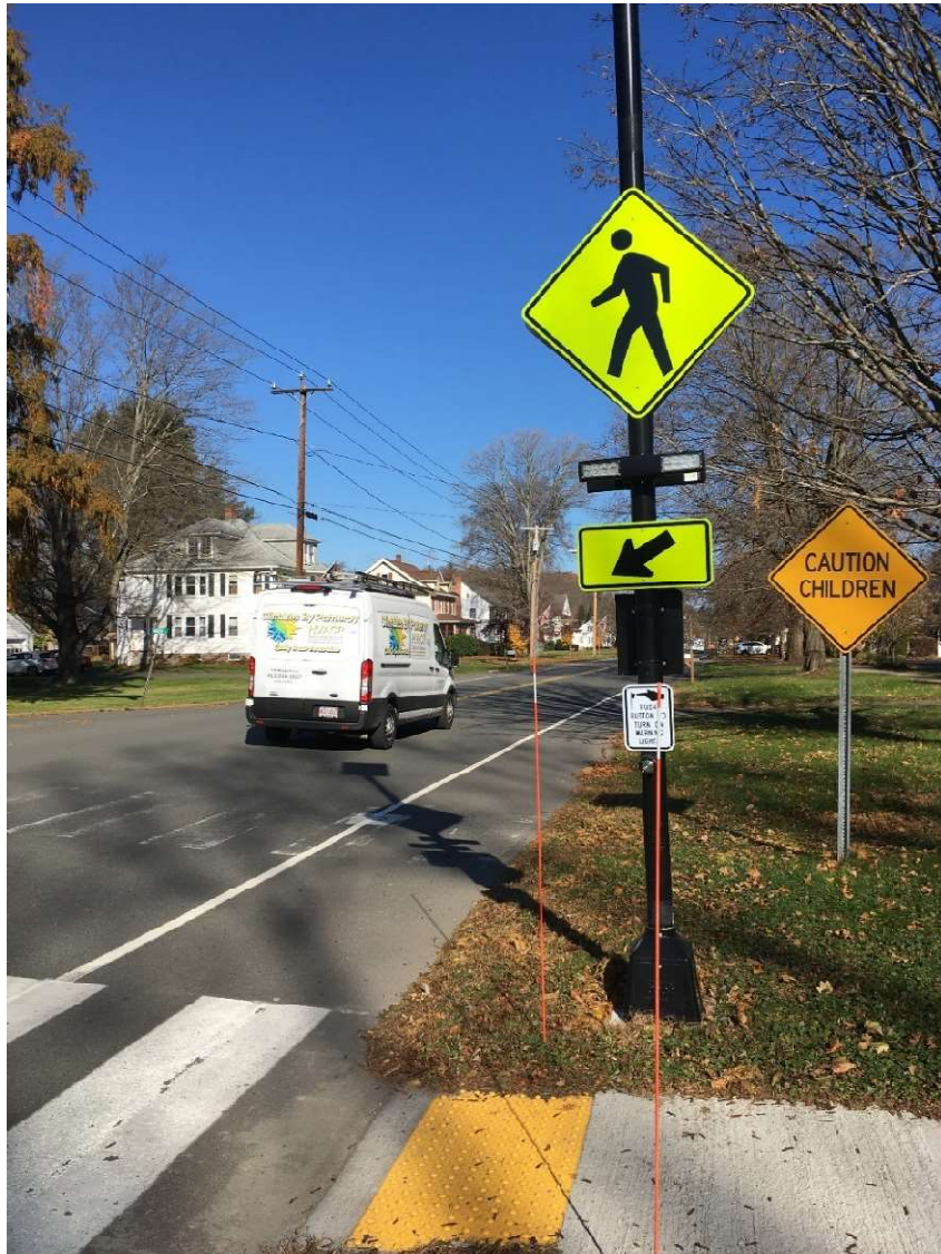
Hatfield DPW installed Rectangular Rapid Flashing Beacons pedestrian actuated signals on the Main Street intersection with North Street in 2023.
